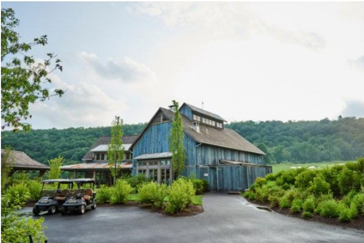
Silo Ridge in Amenia, N.Y. Jeff Lipsky
